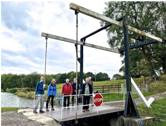
Turflea Lift Bridge - Peak Forest Canal
